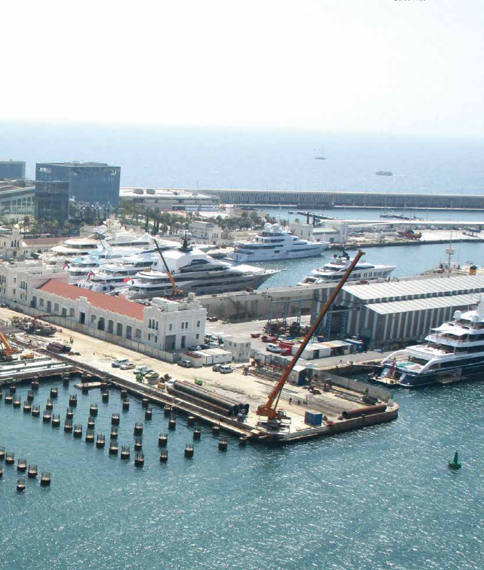
Syncrolift yacht dock, Barcelona Bored Piles
