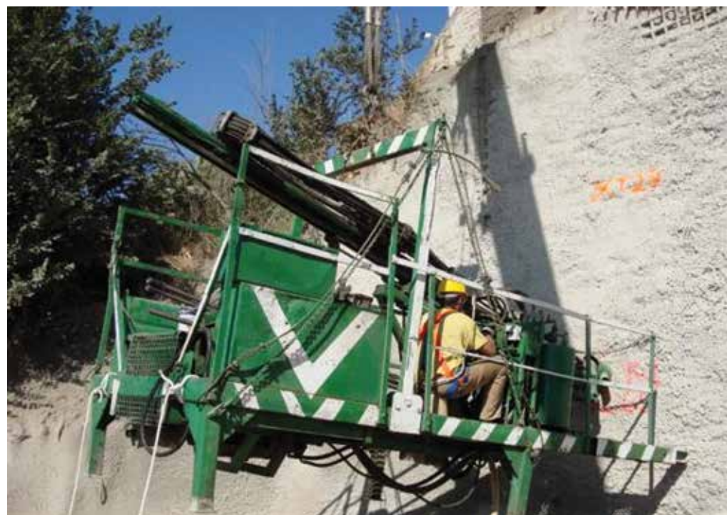
Landslide in Bonares. Huelva, Spain Soil Nailing
