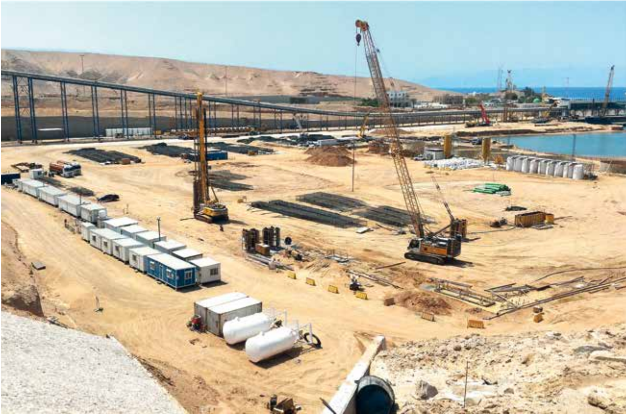
Aqaba New Port Phase II (Jordan) Diaphragm Wall with Hydrofraise
