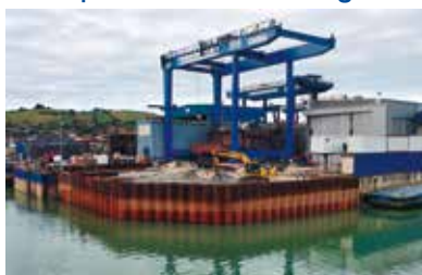
Sheetpiles / Metal Bracing
