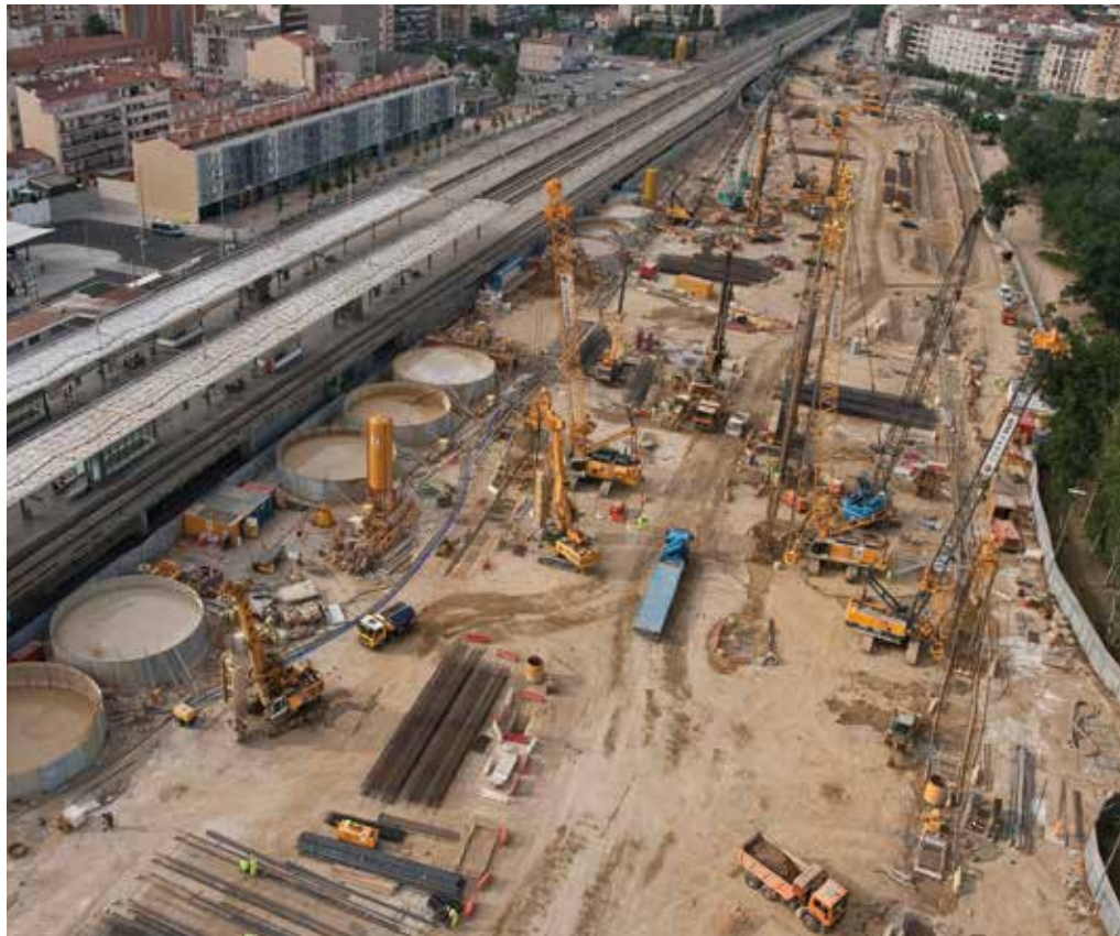
New High-speed railway station. Gerona, Spain Diaphragm walls, Bored Piles, Trench Cutter
