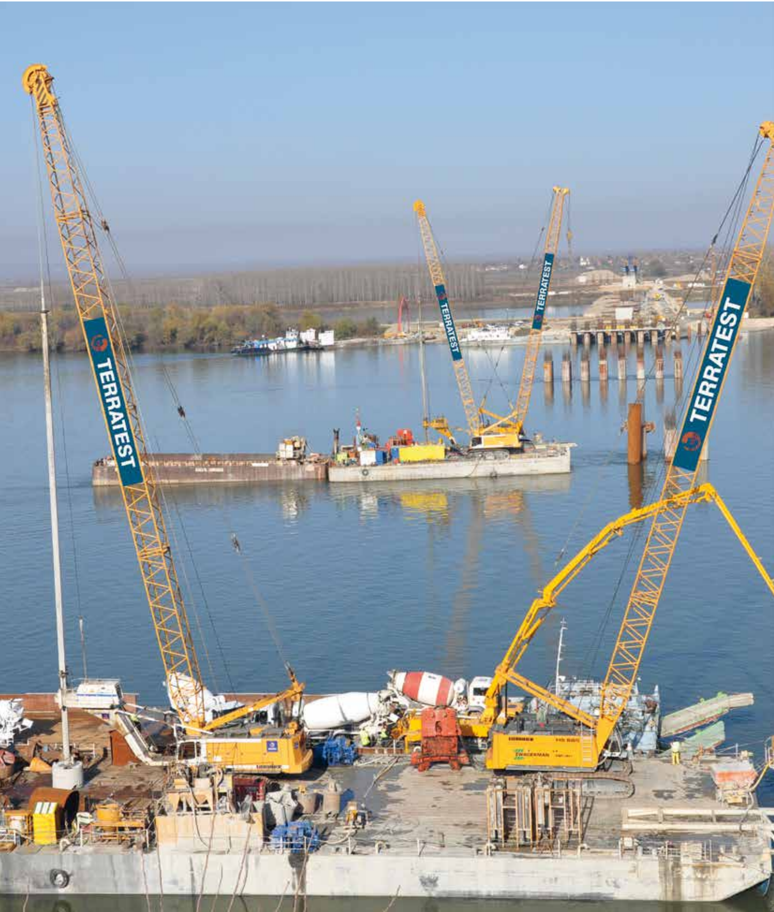
International Bridge over Danube River, connecting the cities Vidin (Bulgaria) and Calafat, Romania Bored Piles
