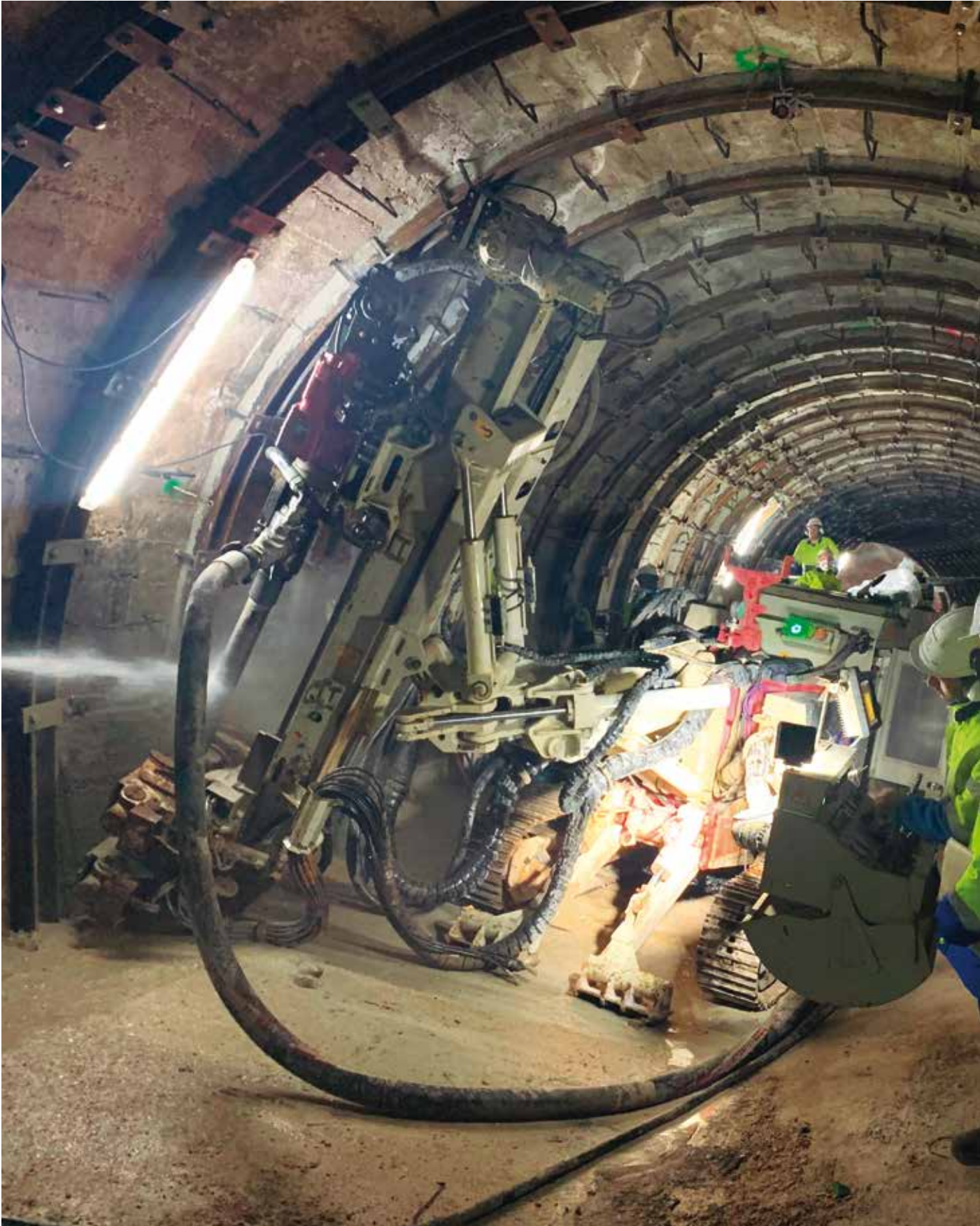
El Sing Ravine, Alcoy Cmpaction Gouting
