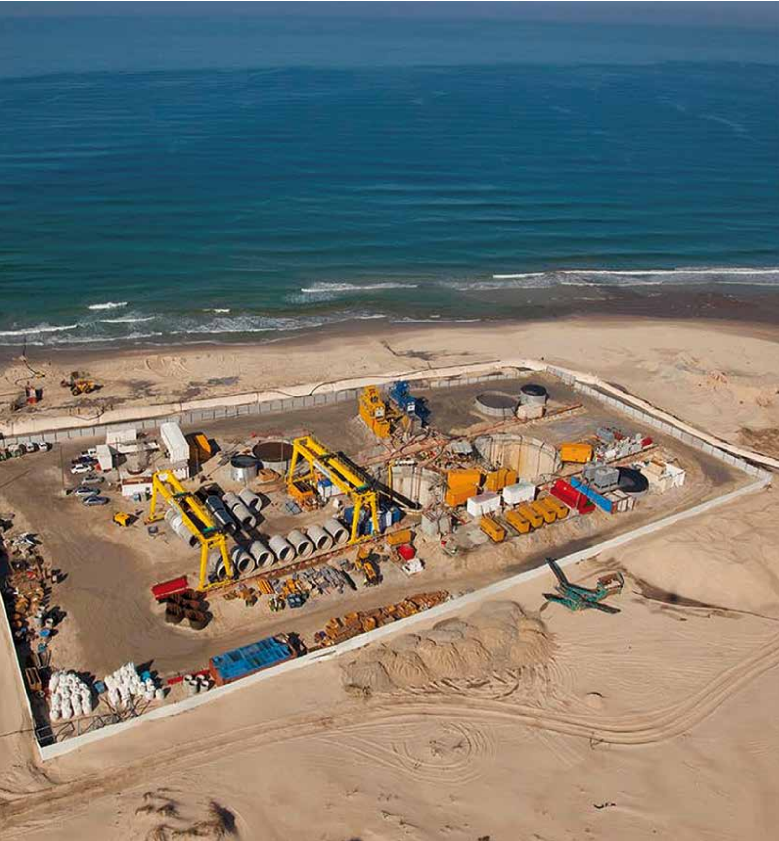
On Shore and off Shore Tunnels. Desalination Plant, Sorek, Israel Tunneling
