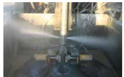
Compensation and Compaction Grouting
