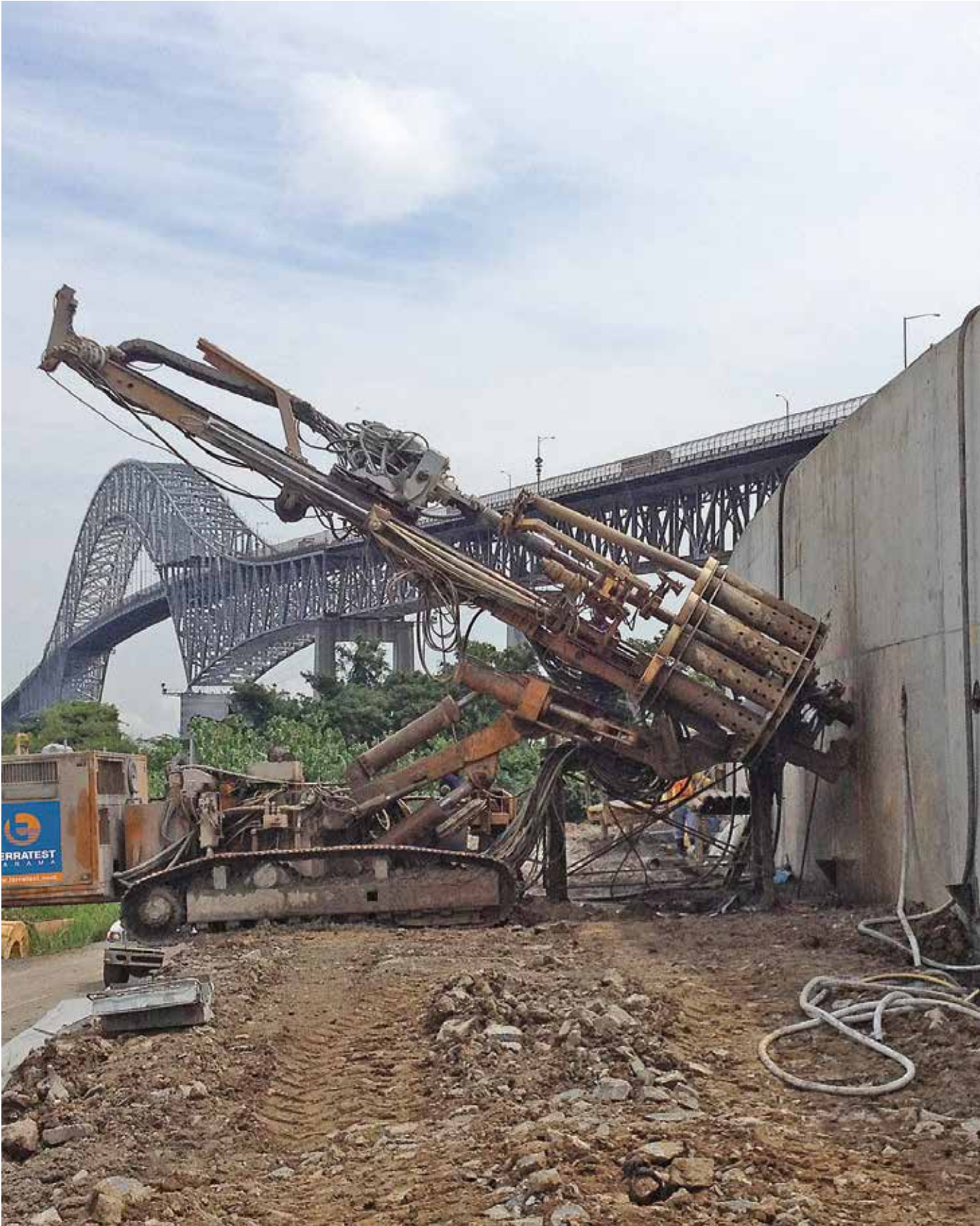
Puente de las Americas Rehabilitation, Panama City, Panama Ground Anchors
