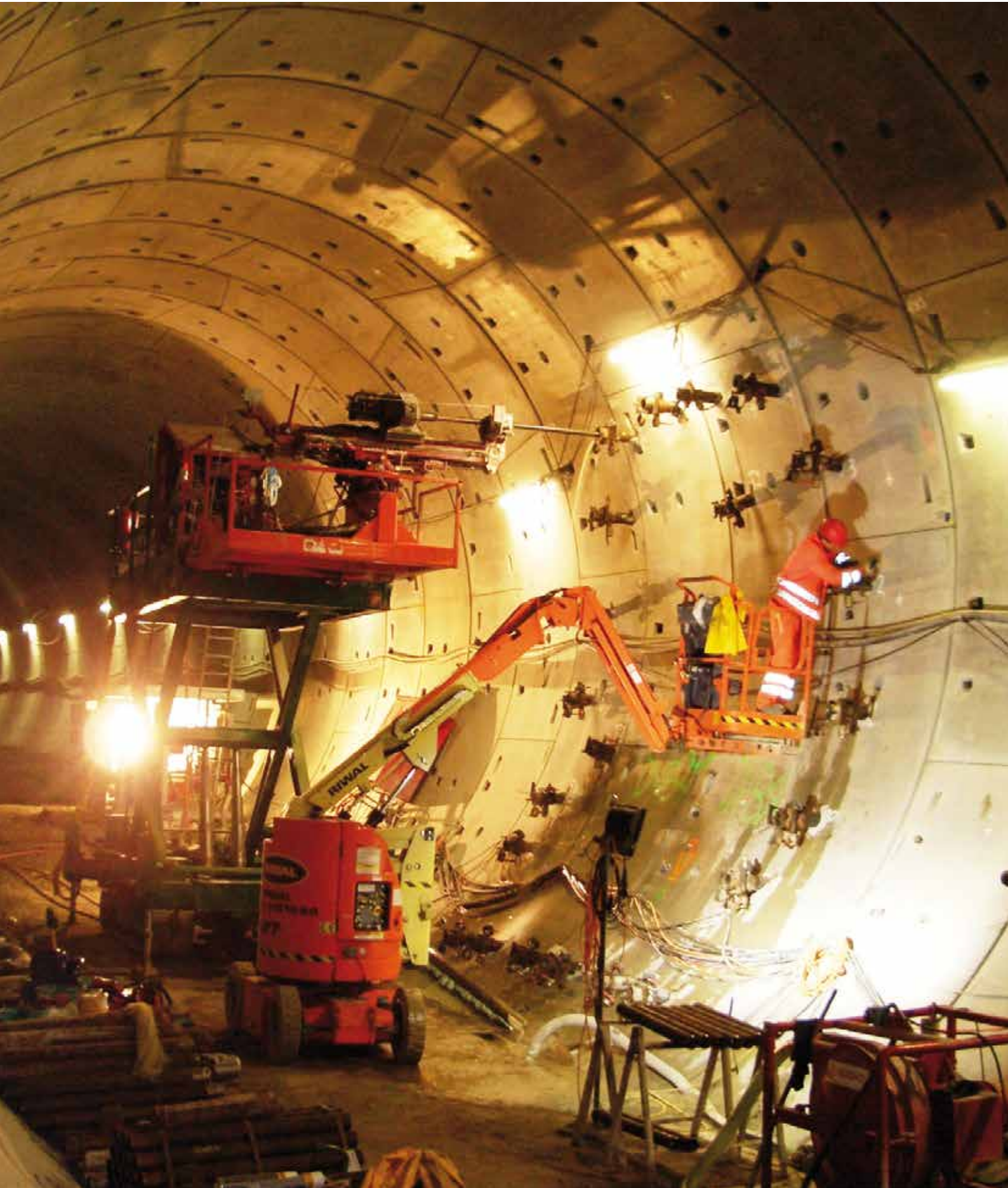
Hubertus Tunnel. La Haya-Amsterdam Motorway, La Haya, Holland Ground Freezing
