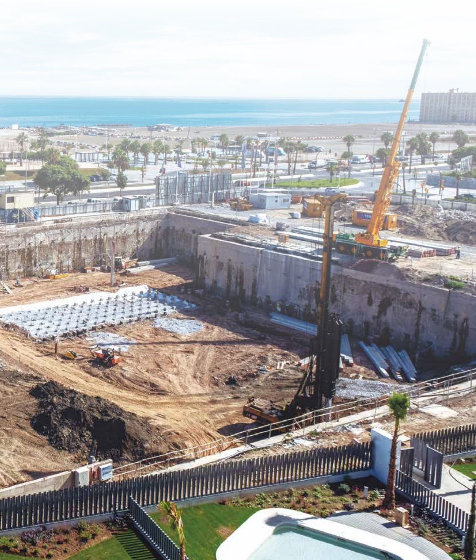
Picasso-Towers, Malaga. Precast Piles and Ground Anchors
