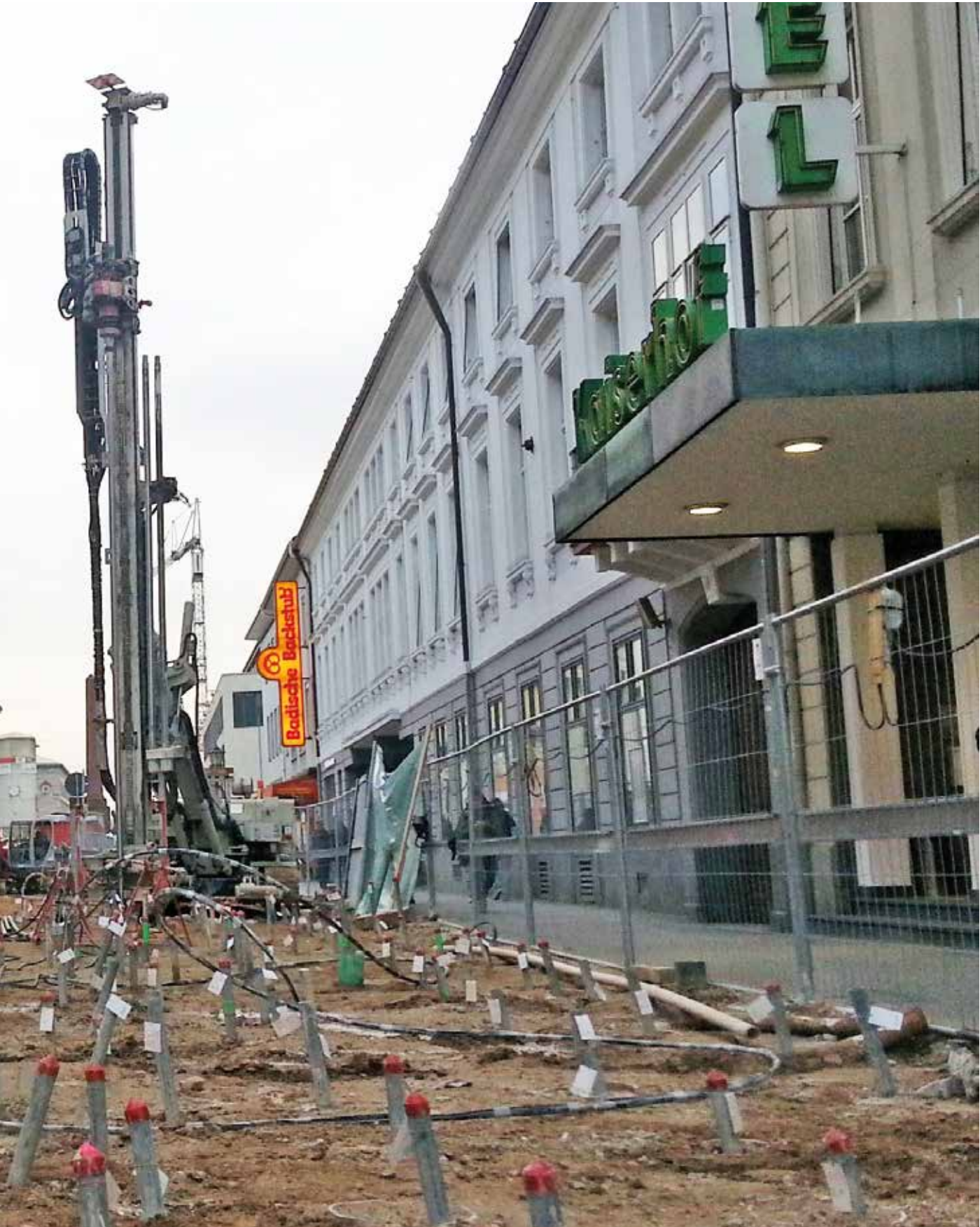
City Metro Tunnel Karlsruhe Manchette Pipe Grouting Grouting
