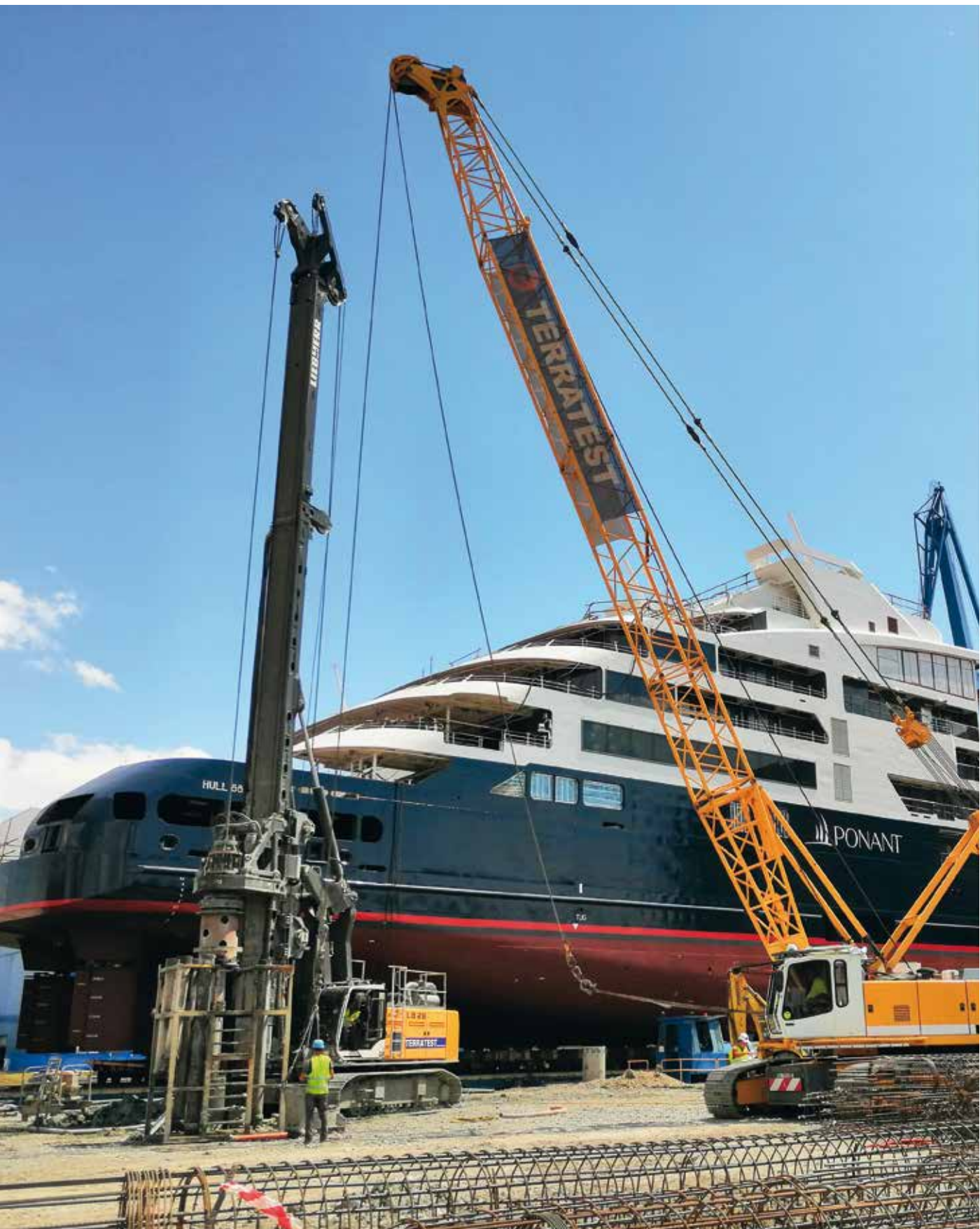
Quay Extension, Tulcea Port, Phase 7, Romania Bored Piles
