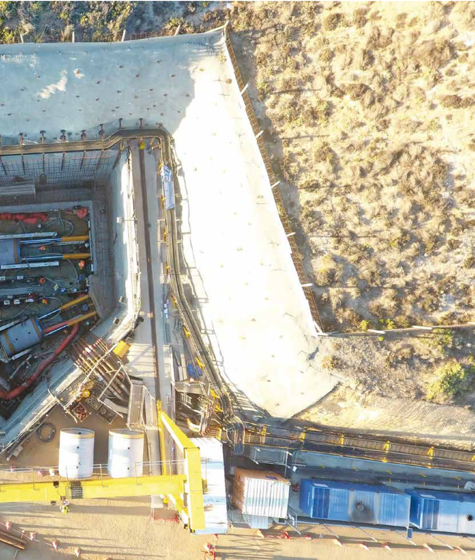
Desalination Plant Los Pelambres, Chile 2 Pipe Jacking drives with Hydrosield AVN 2000; AVN 1800
